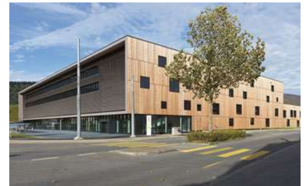
Figure 4-6: Distinctive Material and Form at Entry Area
