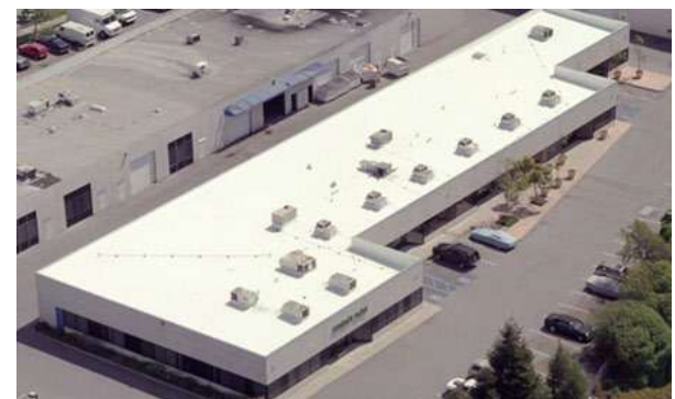
Figure 4-4: White Material on Rooftops
