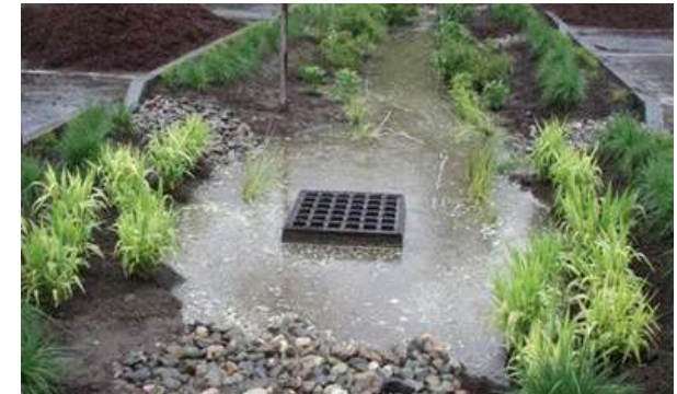
Figure 2-5: Stormwater Bio-Swale Landscaping & Planting
