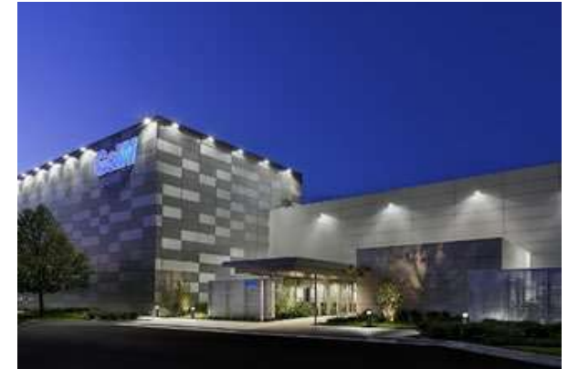
Figure 8-1: Unifying and Aesthetic Lighting Elements
