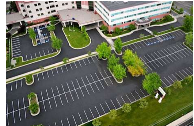
Figure 3-4: Well-Divided Parking Lot
