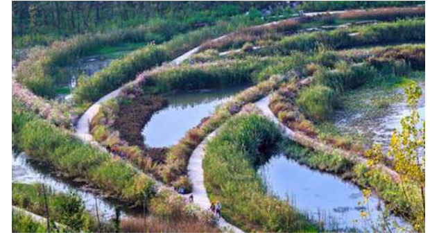
Figure 11-1: Stormwater Retention Ponds
