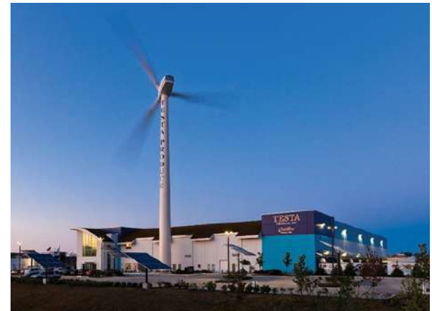
Figure 4-9: Wind Turbine and Solar Panel
