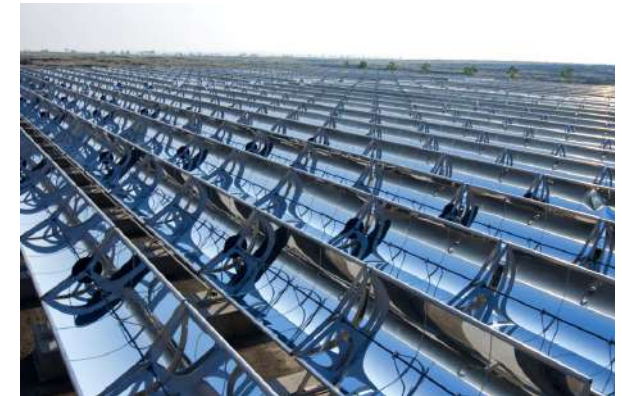
Figure 10-2: Parabolic, Solar Concentrator System.
