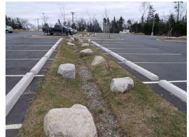
Figure 11-2: Bio-Swale Filters Pollutants from Runoff
