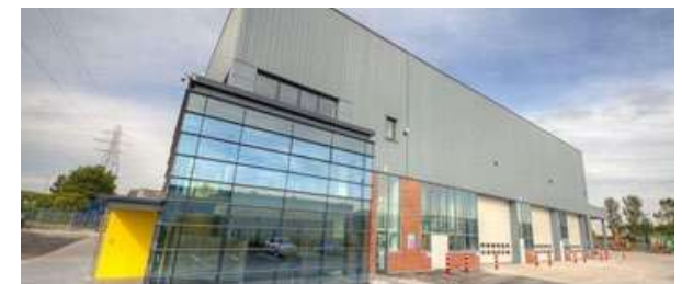
Figure 4-7: Distinctive Material and Form at Entry Area
