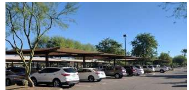
Figure 5-8: Shading Structure Helps To Reduce Heat On The Ground
