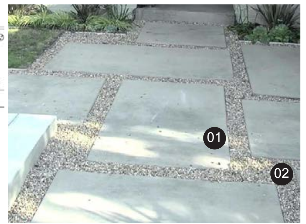
01 800X800MM CONCRETE STEPPING STONE 02 GRAVEL
