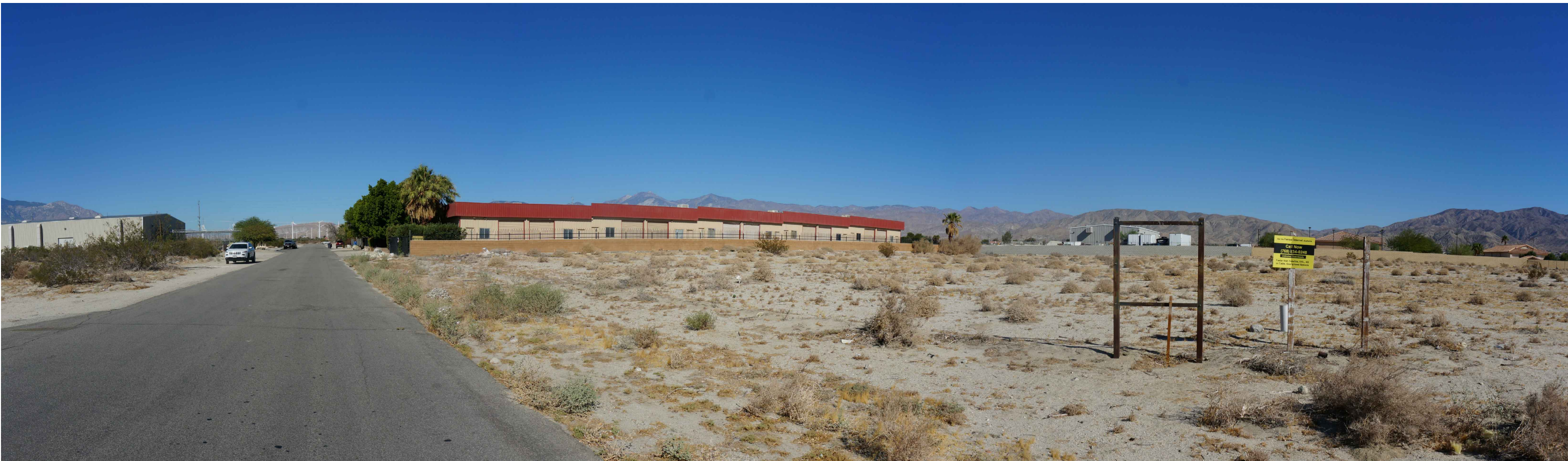
PHOTOGRAPH NO. 4: SOUTH EAST CORNER
